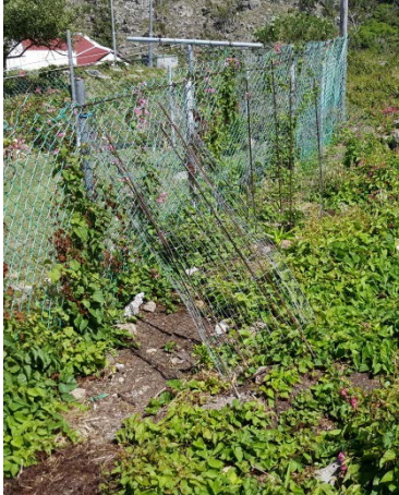
The topped over fence. Picture credit: Judit Planas i Puig
